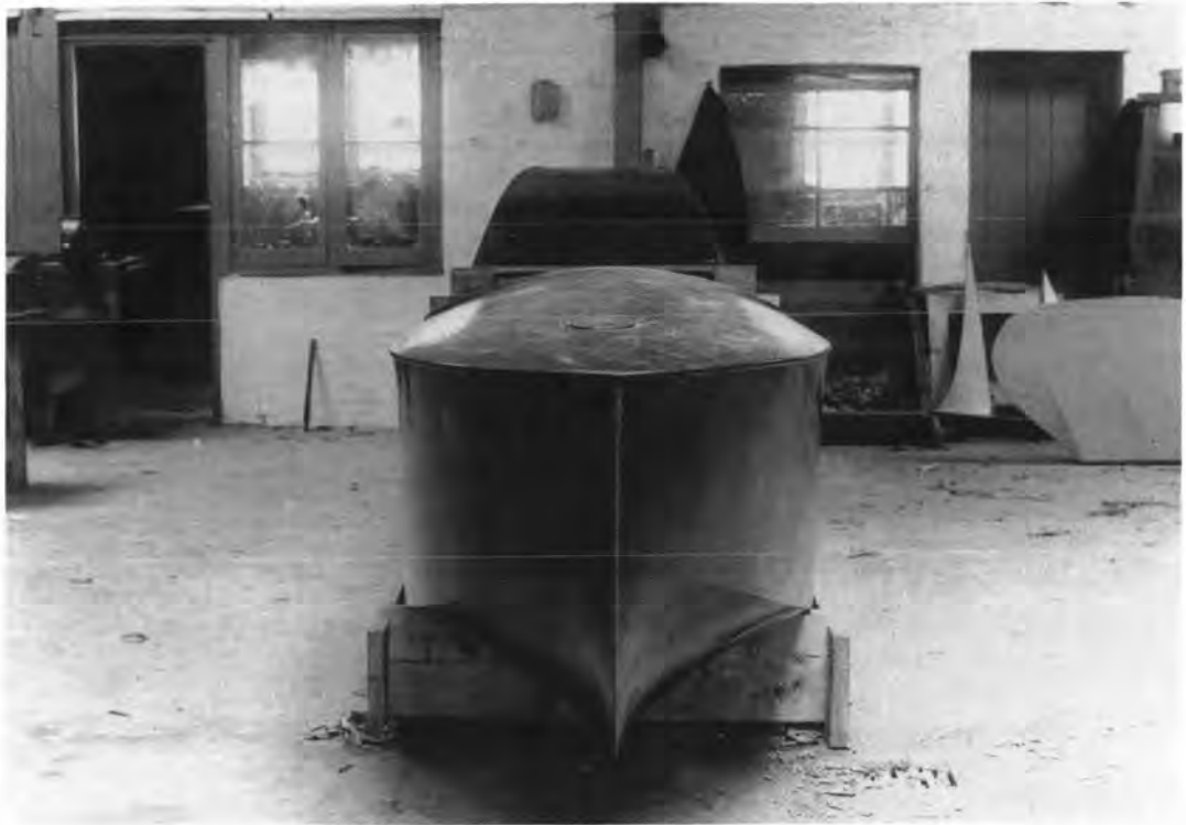
Front of the hull of the Wigram Flying Boat at East Cowes. :Westland Aerospace Ltd — C5606
