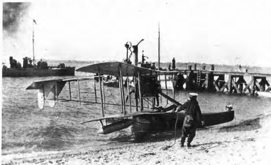
Bat Boat No 118 in mid-1914 with triangular fins and a headlight. It was flown in this form by Lieut J.L. Travers at the Naval Review. :G. Quick
