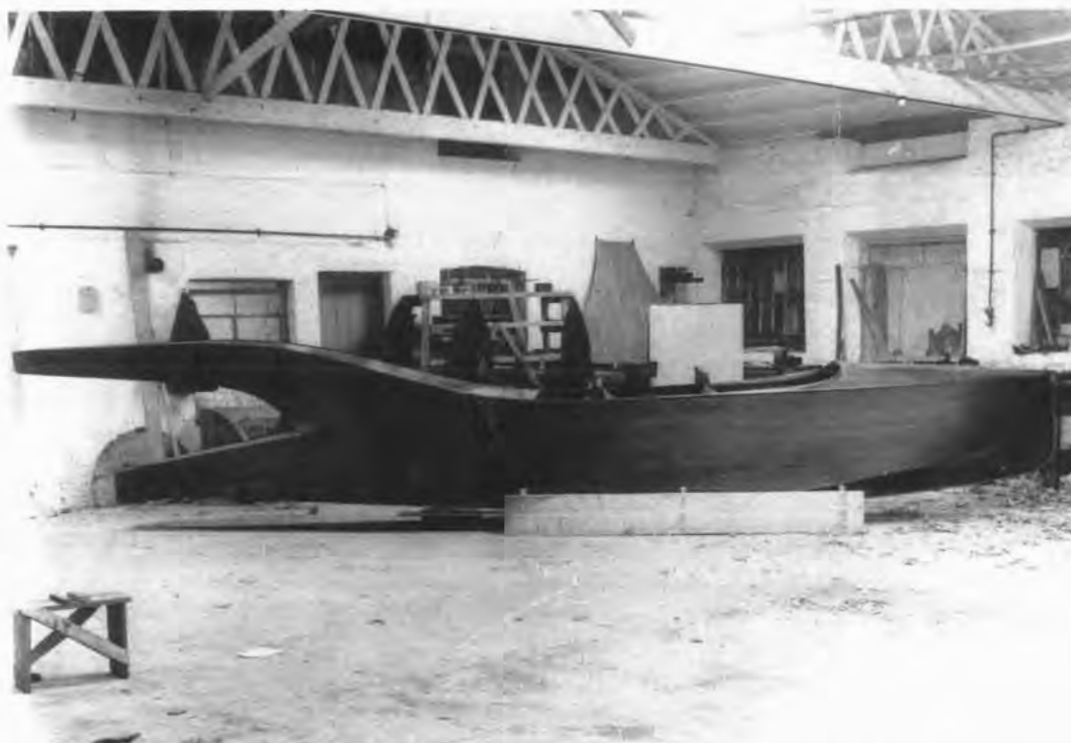
The Wigram Flying Boat under construction in the works of S.E. Saunders Ltd at East Cowes, Isle of Wight. This machine was not completed. :Westland Aerospace Ltd — C5604
