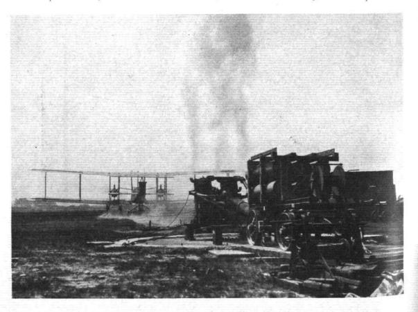
was resumed. Mr. R. Falkland Carey, who had designed the Waygood-Otis catapult, designed a new one, which followed in a general way the lines of the American catapults, with the motion of the ram transmitted to the launching carriage by wire ropes over pulleys. The Carey catapult was designed to launch aircraft up to 7,000 lb. weight, the run being 34ft. and the speed 45 m.p.h. The mean acceleration was 2 g. Compressed air was used.
