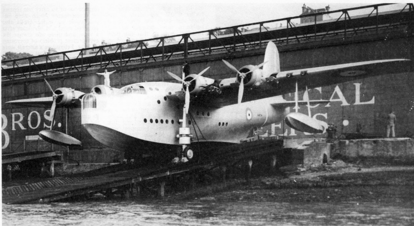
An excellent pre-war picture of the prototype Sunderland outside the Short Bros works at Rochester on its beaching trolley during preliminary engine runs. Note that there are slight differences between the main legs and those shown below.
